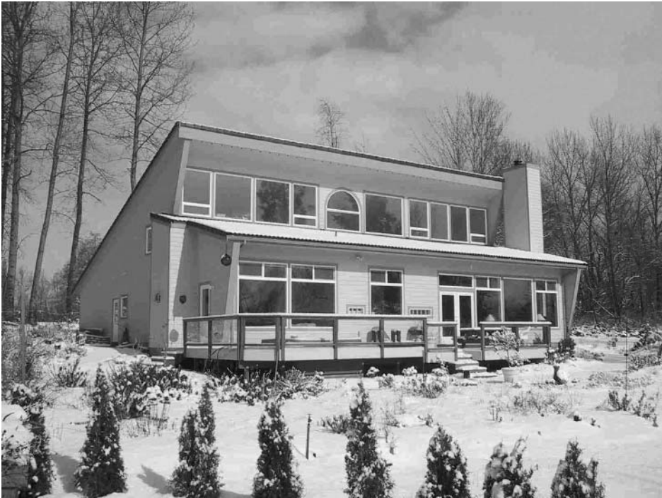
Fig. 11.3 A passive solar home located in Western Washington State, USA, at about 48^{\circ}\text{N} latitude. The annual cost for supplemental (nonsolar) energy in this cloudy and rainy location is less than $150 (Photo by author).
