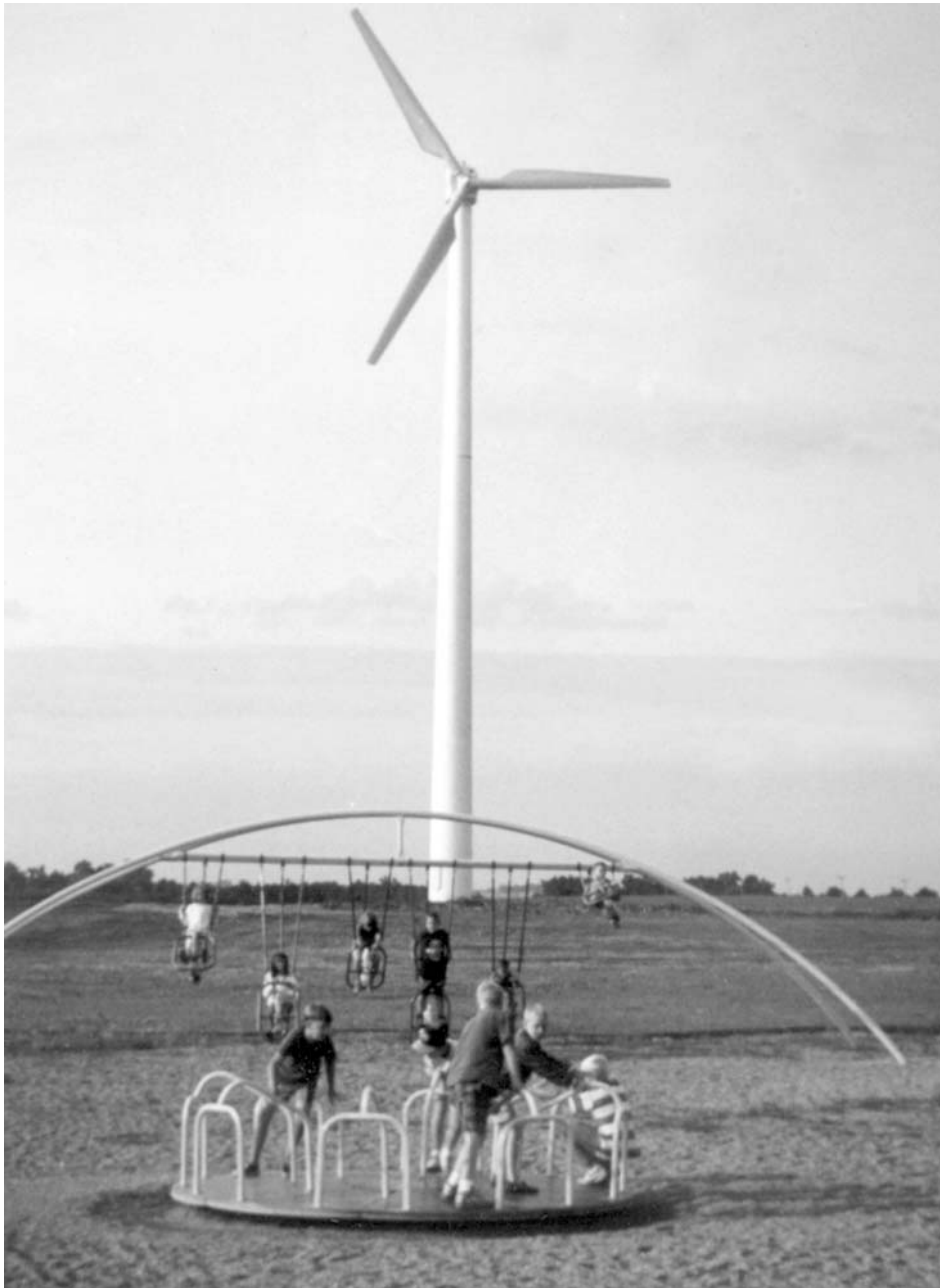
Fig. 11.2 A 250-kW turbine installed at the elementary school in Spirit Lake, Iowa, provides an average of 350,000 kWh of electricity per year, more than is necessary for the 4,900 m 2 (53,000 ft 2 ) school. Excess electricity fed into the local utility system has earned the school $25,000 over five years. The school uses electricity from the utility at times when the wind does not blow (Courtesy AWEA 2002. American Wind Energy Association . 122C Street NW, Washington DC 2001. Available from: http://www.awea.org ).
